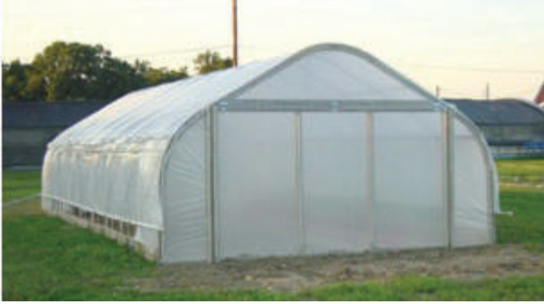
Figure 4.7: High Tunnel (Rutgers University, 2003).
